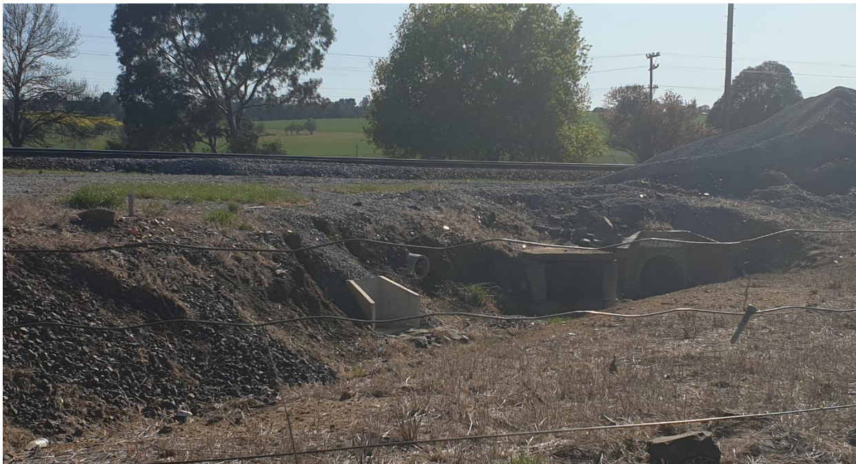
Photo 18: Obstructed Stormwater Inlet near Whitton Lane at Short Street
