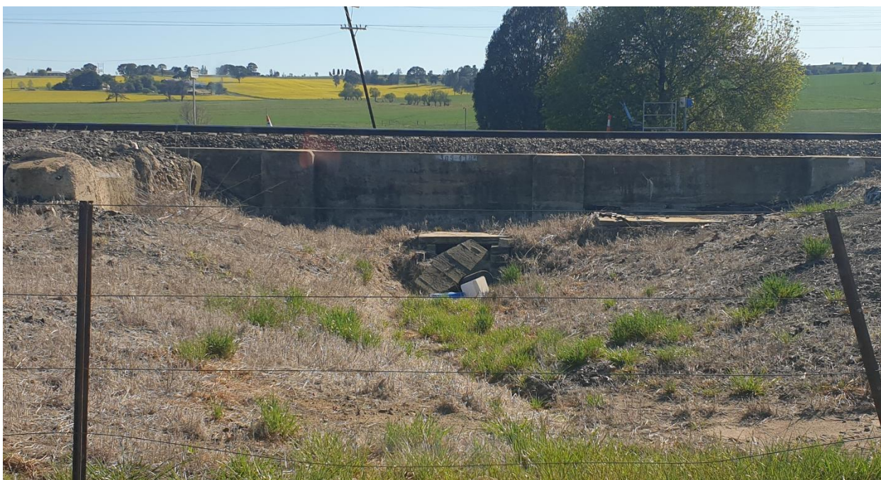
Photo 18: Obstructed Stormwater Inlet near Whitton Lane at Short Street
