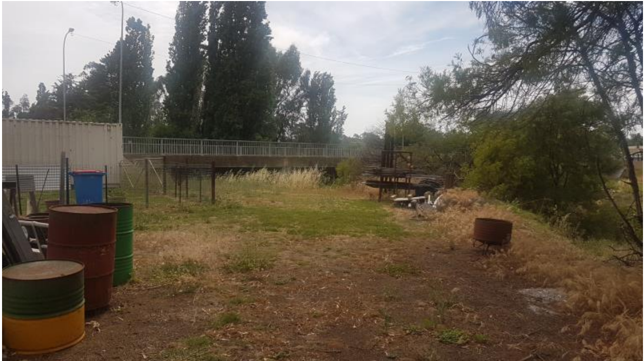
Photo 7: Indicative Levee Location behind Metalcraft Shop
