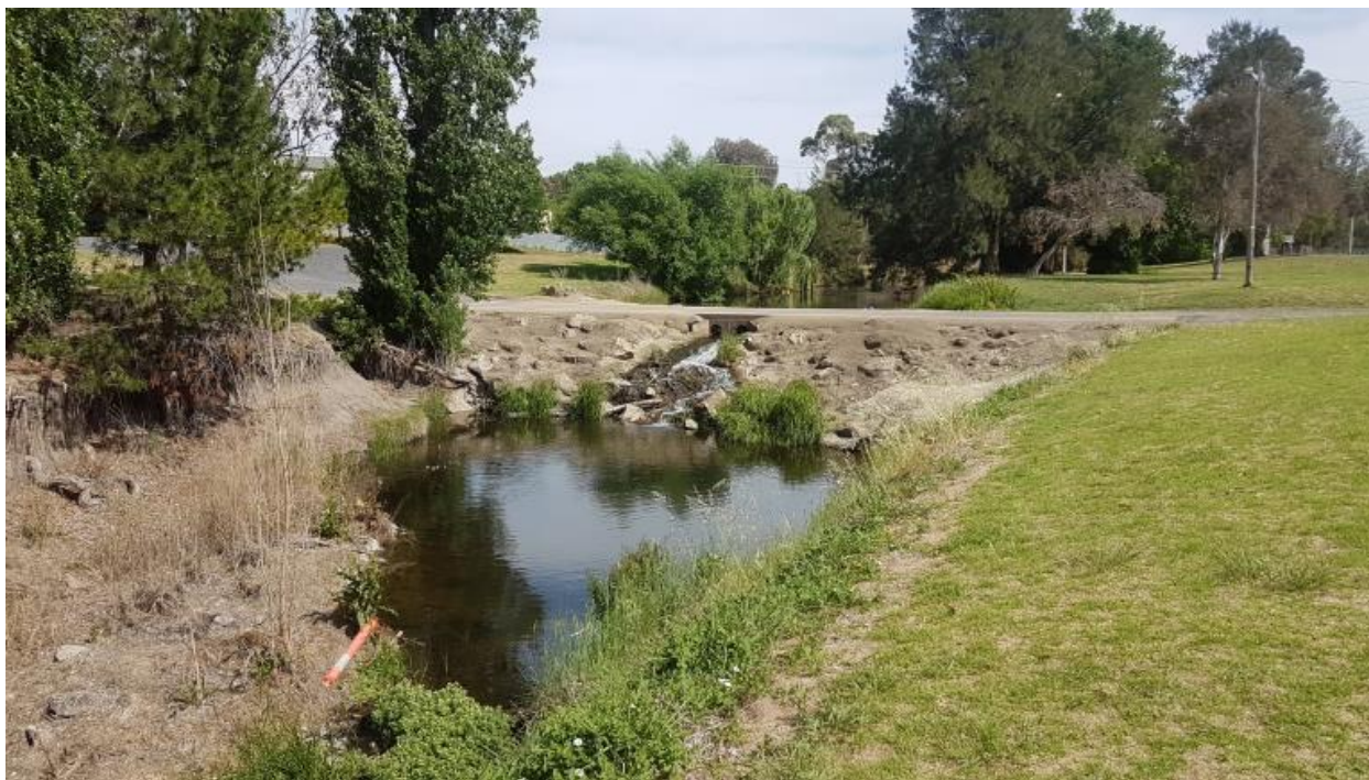
Photo 11: Neill Street Causeway (November 2018)
