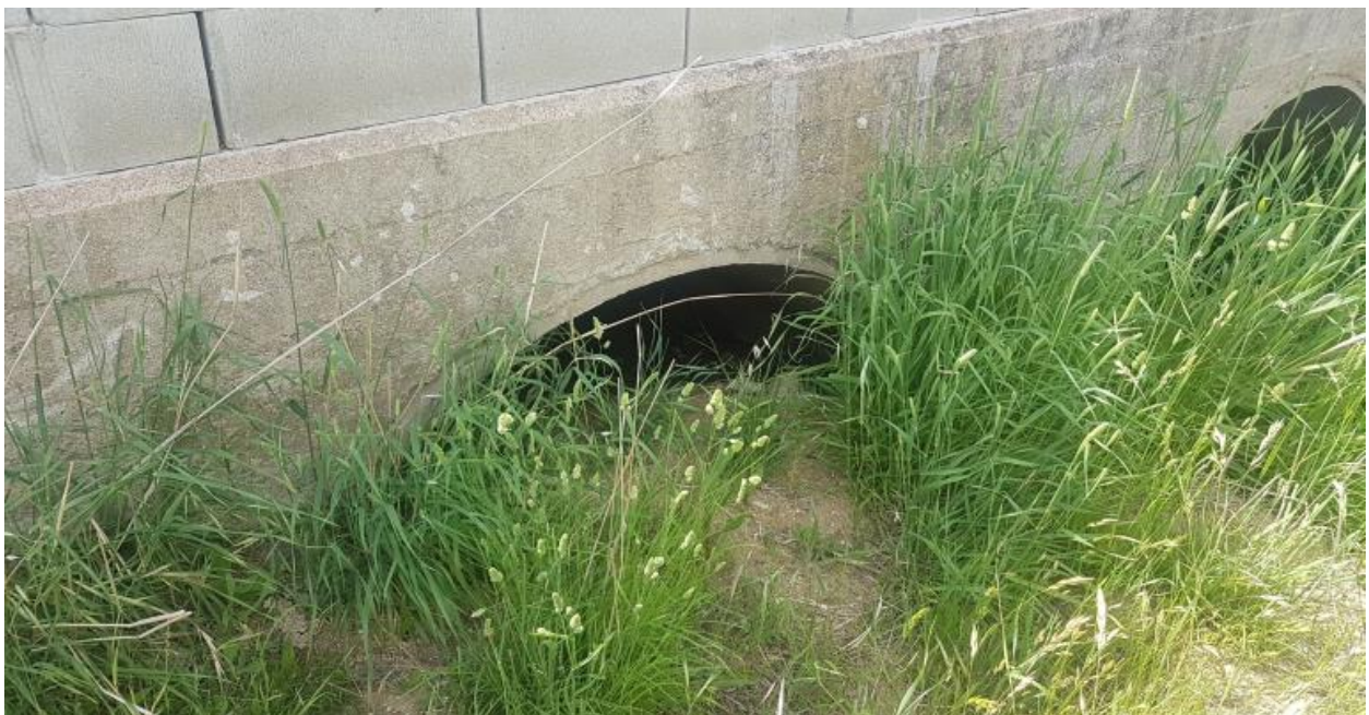
Photo 20: Blockage at Aurville Road Culverts (November 2018)
