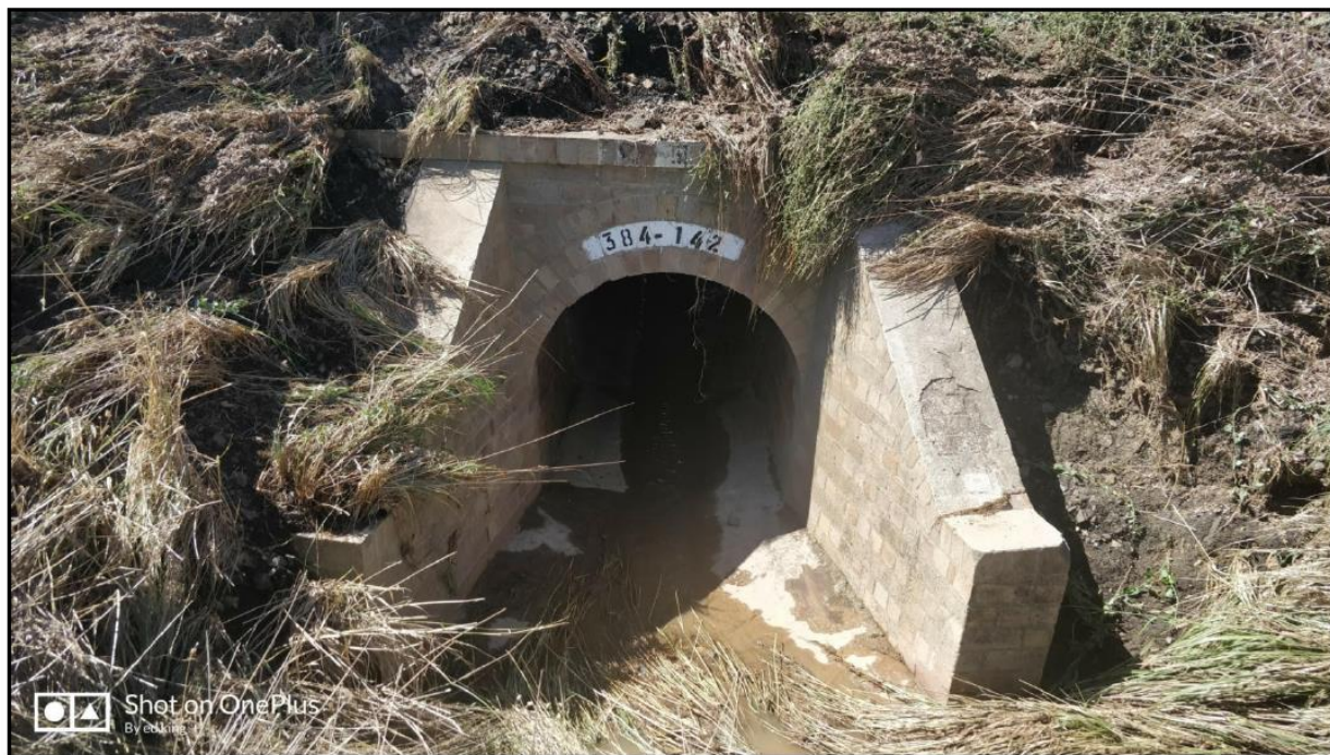
Diagram 4: Cunningham Plains Creek Constriction at Railway Culvert
