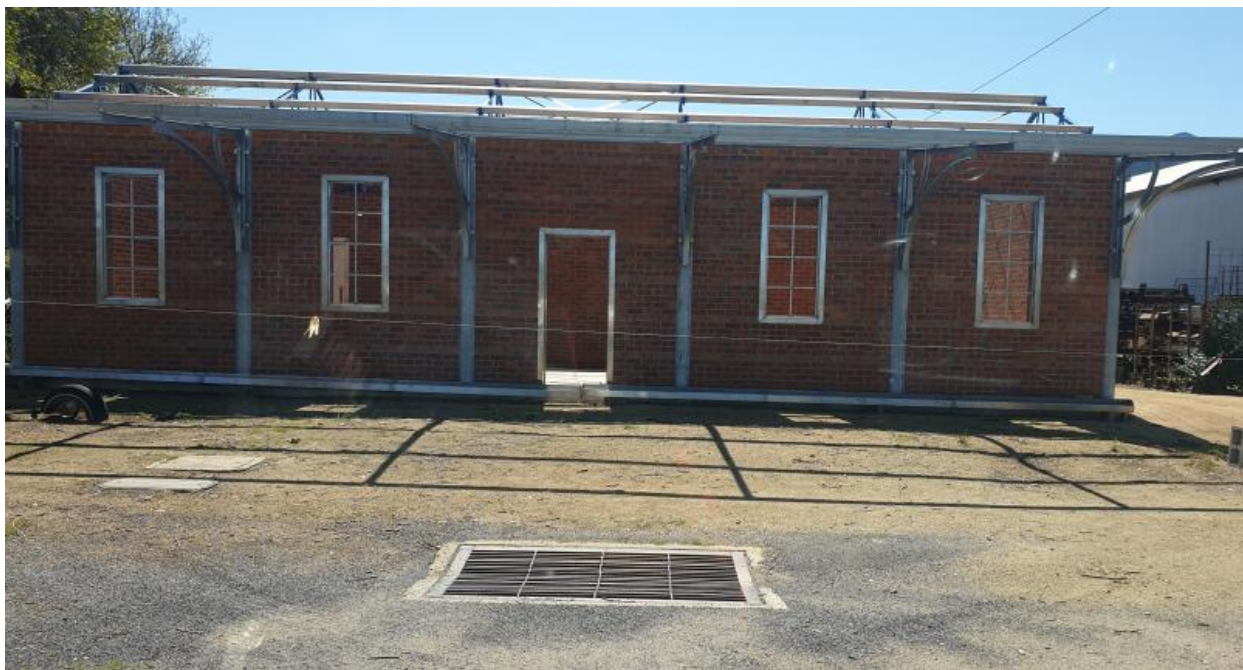
Photo 16: New Building at 371 Albury Street (September 2019 – Site Visit)
