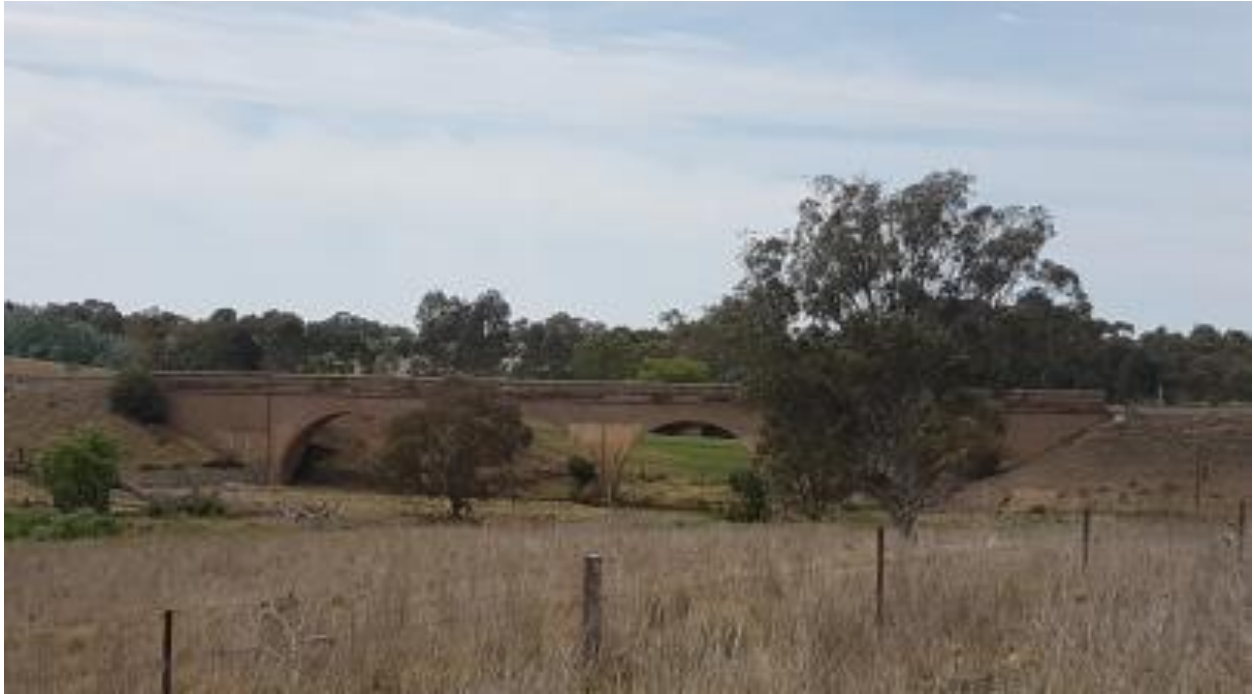
Photo 9: Railway Arch Bridge on Currawong Creek
