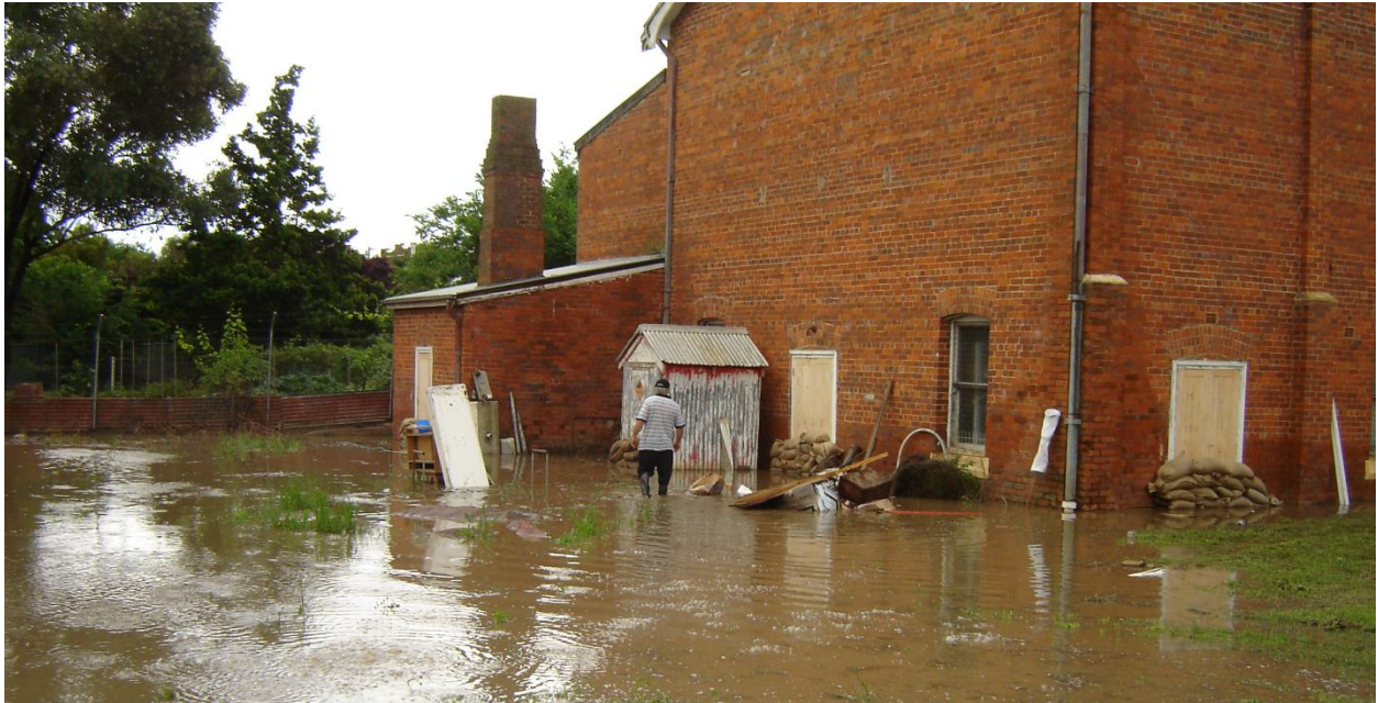
Photo 21: Flooding at Museum in December 2010
