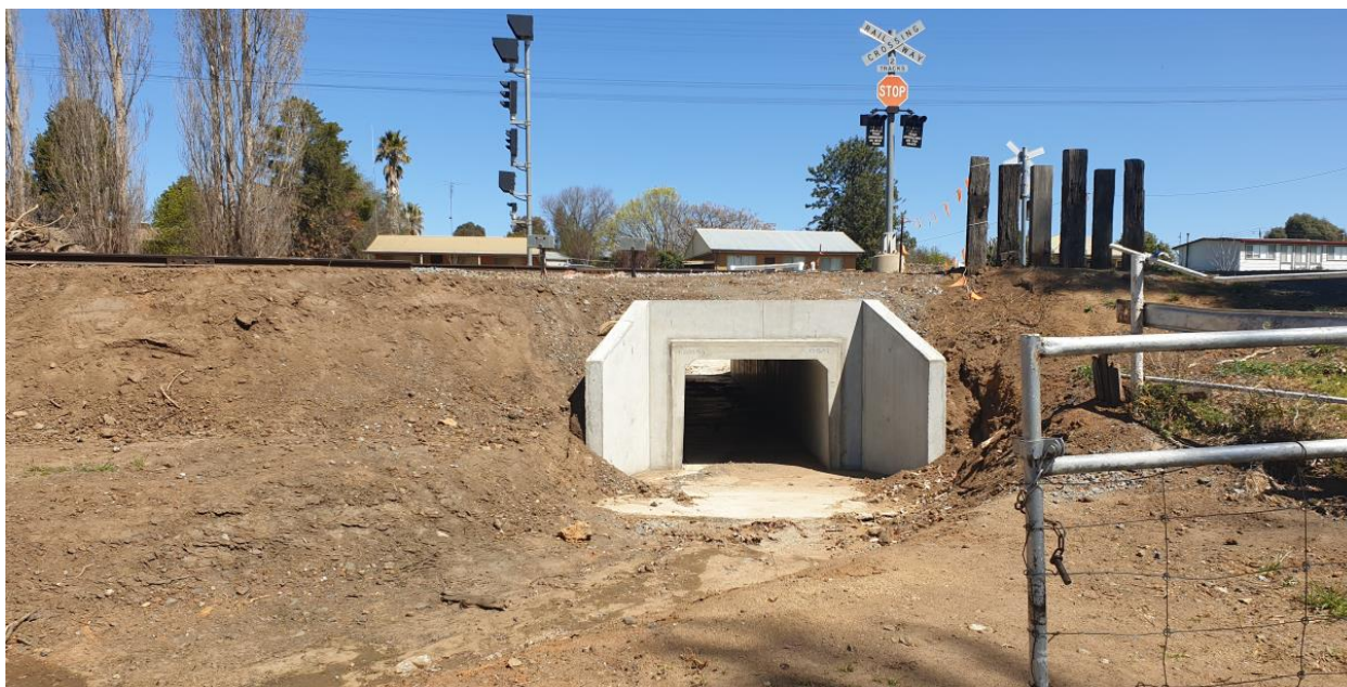
Photo 19: Upgraded Railway Culvert near Spacky Lodge
